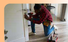
Facilities Manager replacing a lock
